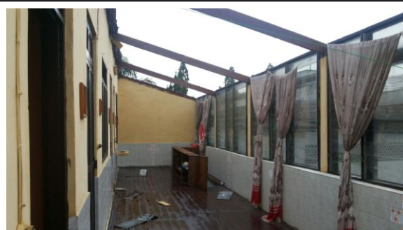
The roof of sitting room upstairs ripped off
